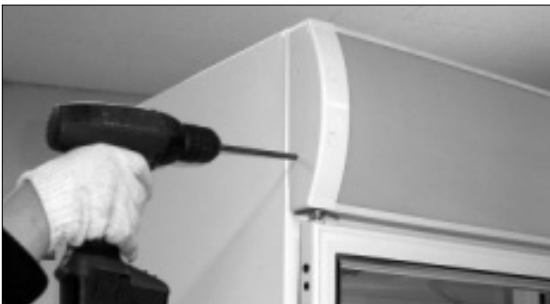
1. Unscrew the left sign frame.
