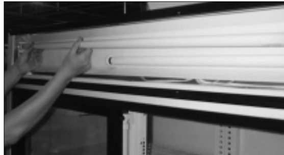
4. Separate the Lamp out of the Lamp Holder and replace it.
