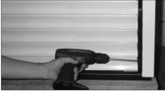
1. Unscrew four screws securing the Bottom Grill.
