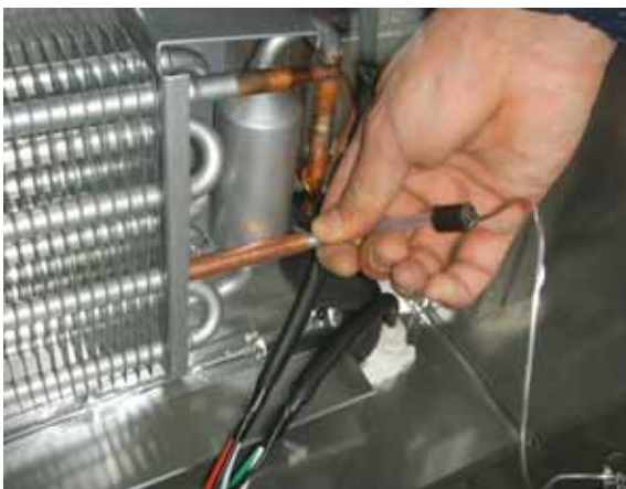
TEMPERATURE CONTROL & EVAPORATOR
